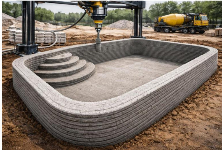
Fig.1. 3D printing of Swimming Tank.
