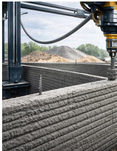
Fig.1. 3D printing of Wall.
