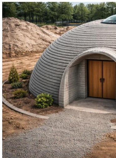
Fig.1. 3D printing of Dome.
