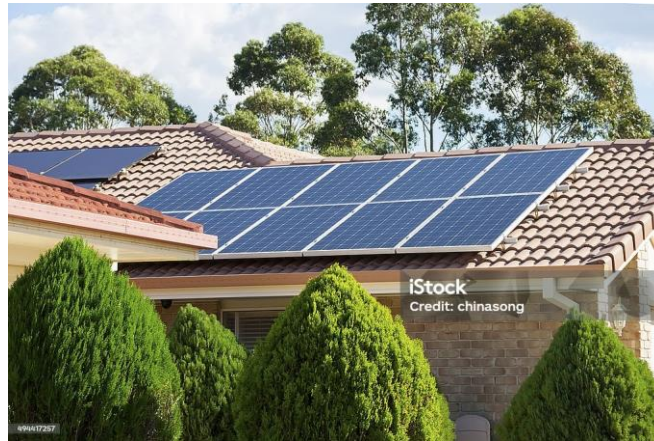
Figure 1: solar-powered residential buildings. ( https://www.istockphoto.com/ )
